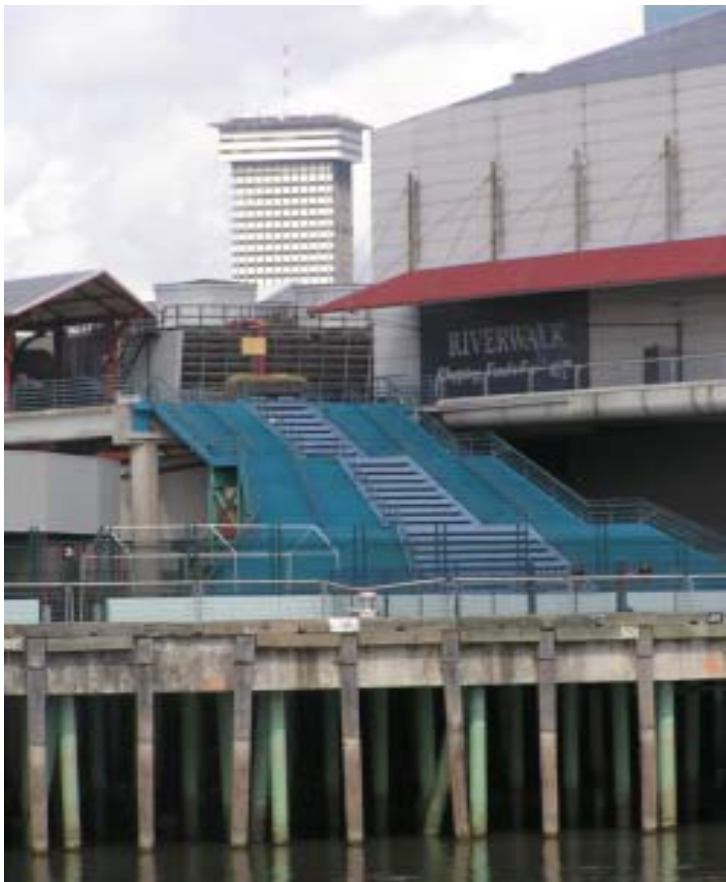
Water Steps at leading from Julia Street Cruise Terminal to balcony walkway and bridge to Convention Center
