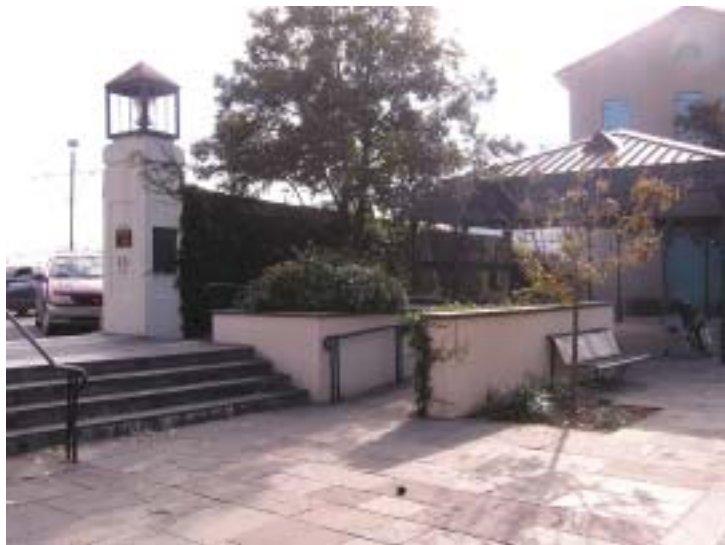
St. Philip Street / French Market floodwall opening
