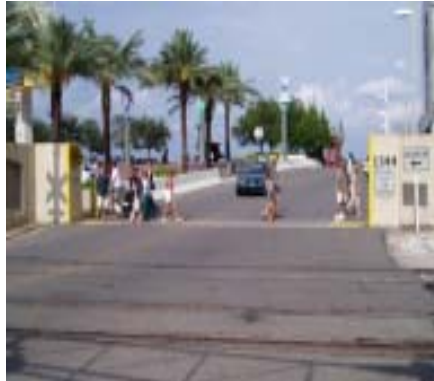
Floodwall opening at Canal Street Ferry Terminal
