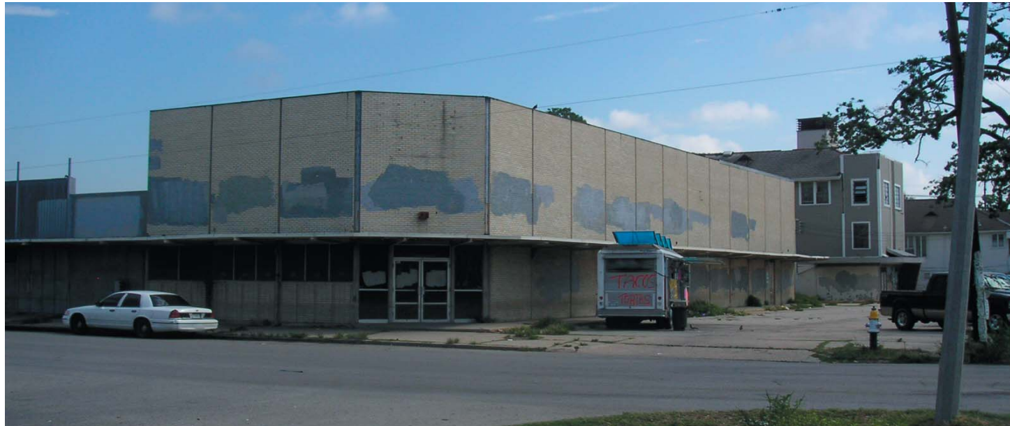
Existing Conditions Photo (Canal Villere)
